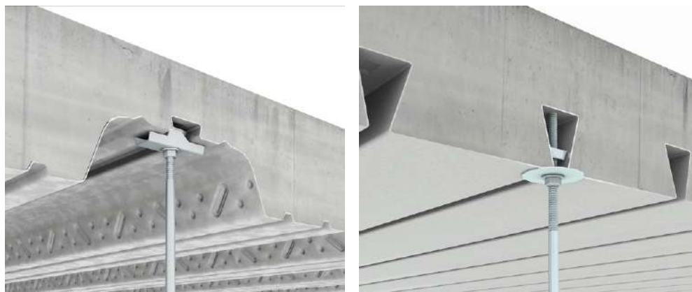
Figure 4.20 Examples of wedge attachment fixings for ceilings and services
