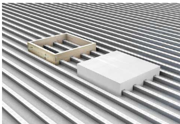
Figure 4.12 Typical examples of boxing out openings
