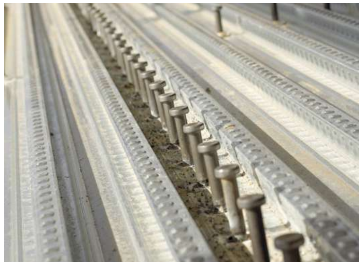
Figure 5.8 A run of stud shear connectors
