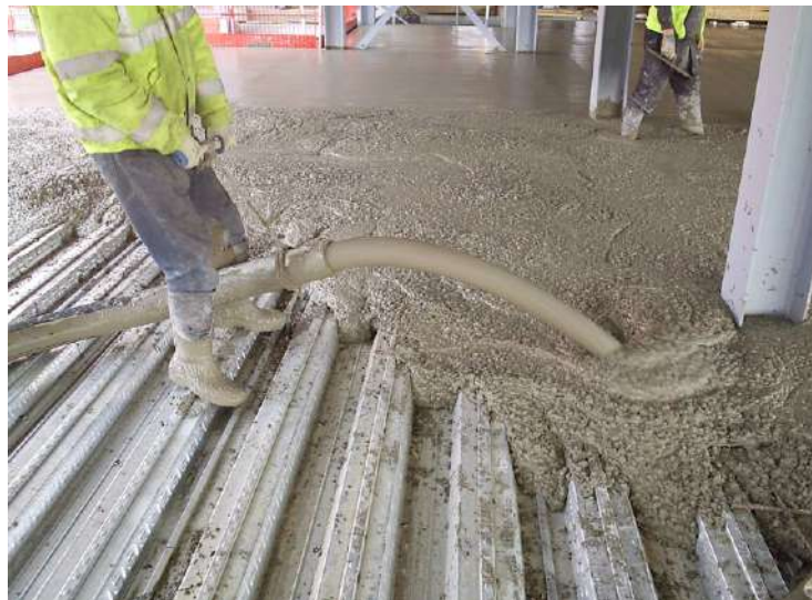
Figure 6.4 Pumping of fibre-reinforced concrete
